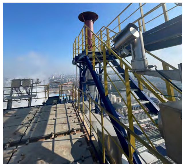
粉煤加压及输送废气新建2根80m高排气筒 (DA092、DA093)
